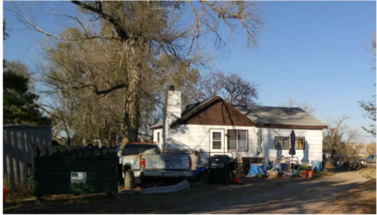
Figure 4. Main building at 6163 East County Road 18
